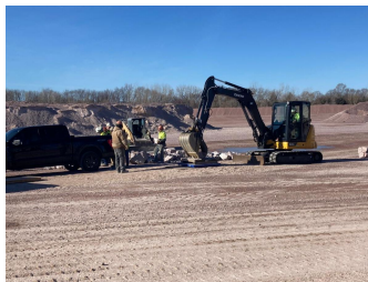
Rip Rap gradation with LGE employees, contractor, and the USACE
